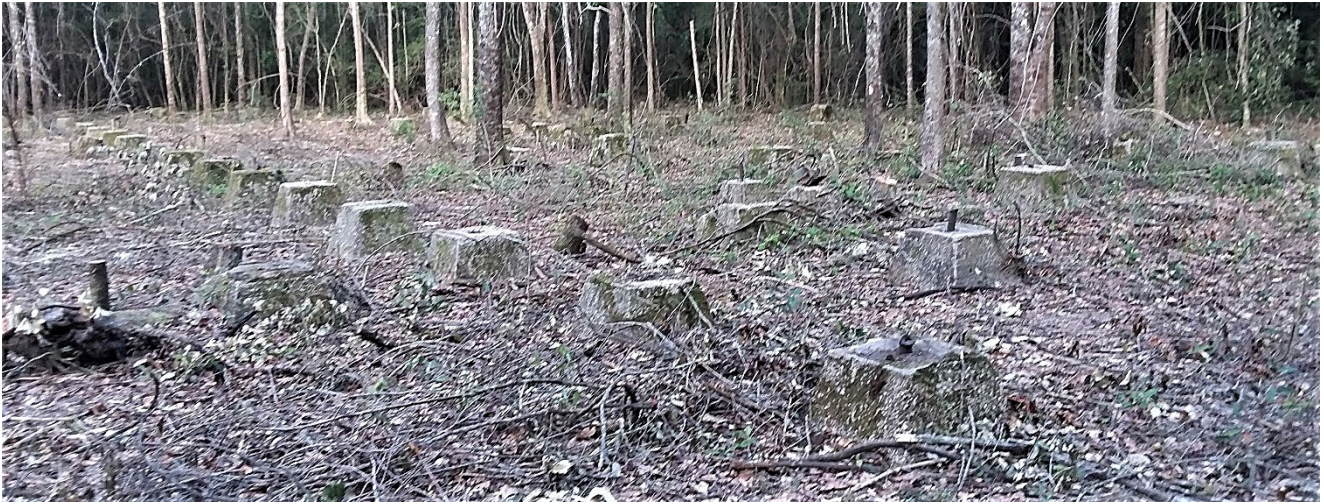
Concrete foundation piers of an unidentified building once standing on Florala Saw Mill Company site at Ghentsville Park in Paxton. Photo by Bruce Cosson, July 2021.
