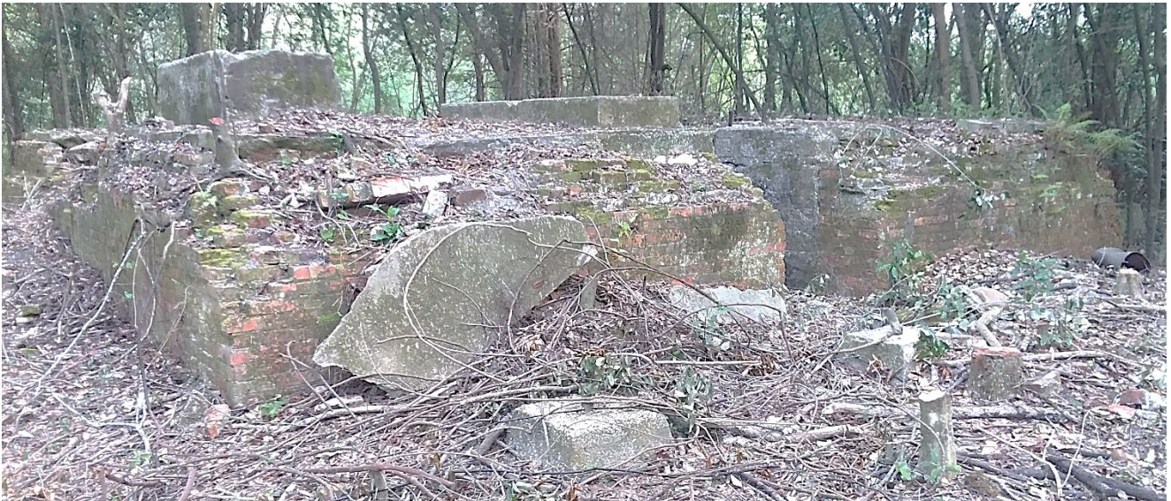
More unidentified building foundations on Florala Saw Mill Company site at Ghentsville Park. Photo by Bruce Cosson, July 2021.
